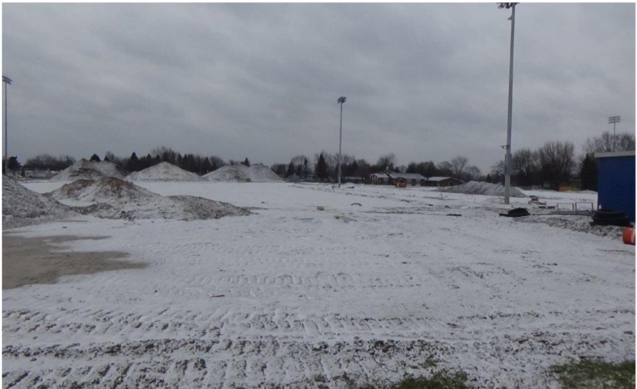
Site Work is on-going as weather permits
