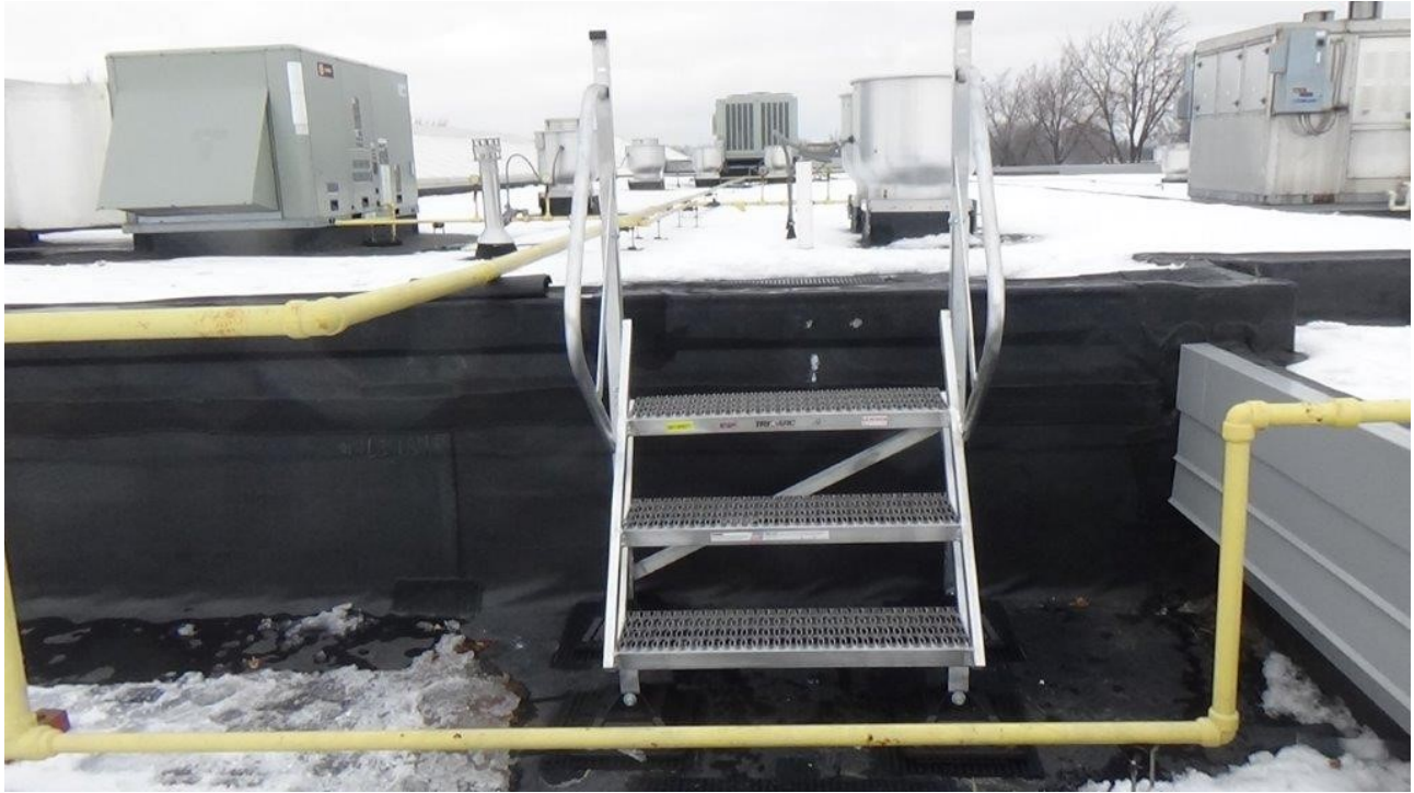
Stairs installed on High School Roof
