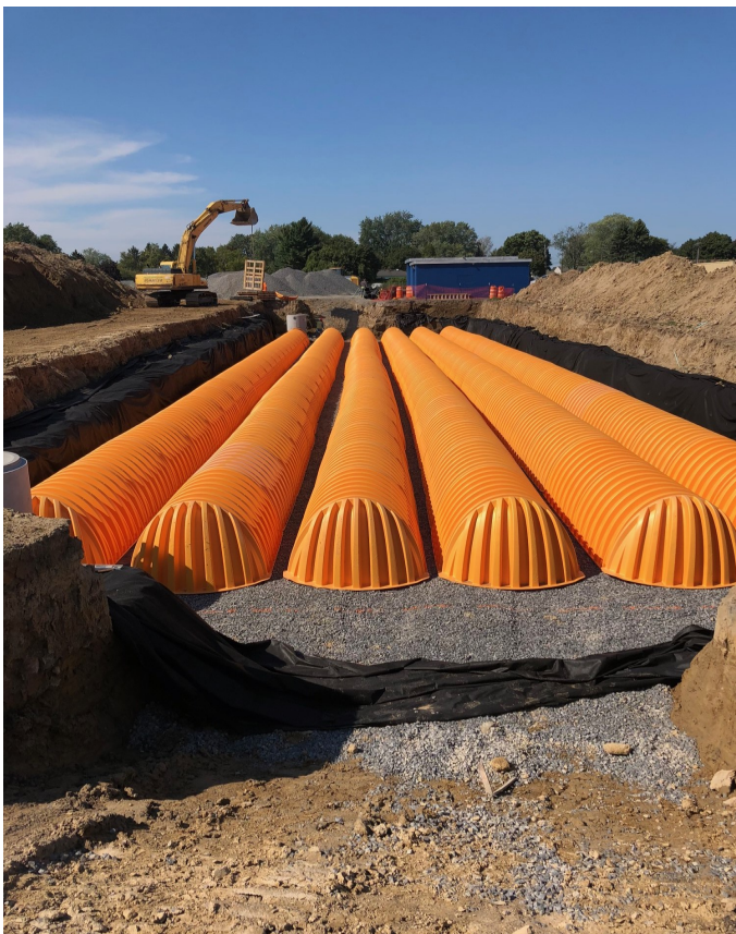
Stormwater System Installation
